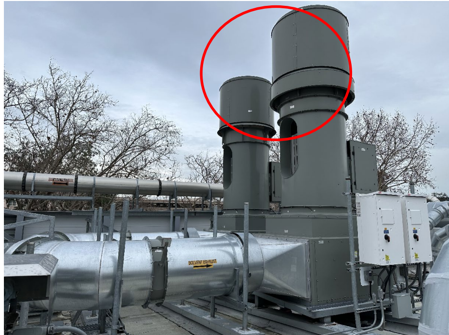
Photograph 11c (IMG_5591.JPG - 01/16/24): A photo of Apple's solvent exhaust piping connecting to one of the main general exhaust systems on the roof of Building 1. The general exhaust system vents the air directly to the atmosphere.
