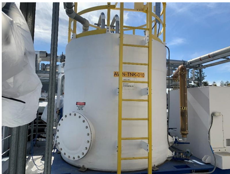
Equalization Tank (AWN-TNK-010)
