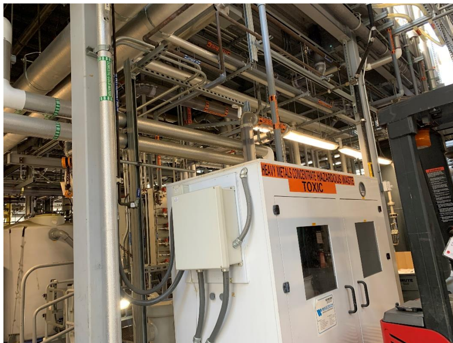
Heavy Metals Concentrate Collection Cabinet (HMC-CC)
